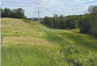
In the photos above, the left shows a portion of the NYES corridor as our crews prepared to remove the existing lattice structures. On the right is the same location today with the new monopoles in place and site restoration underway.
